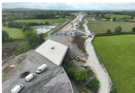
River Bridge M21-C3
