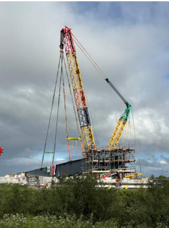
RVB04 River Bridge Steel Beam Lift
