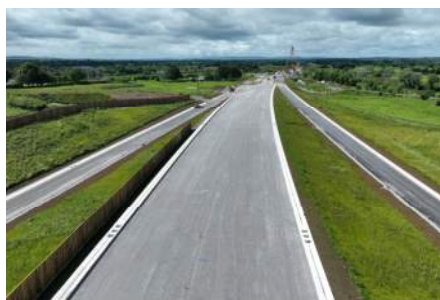
Adare Junction – ready for Pavement
