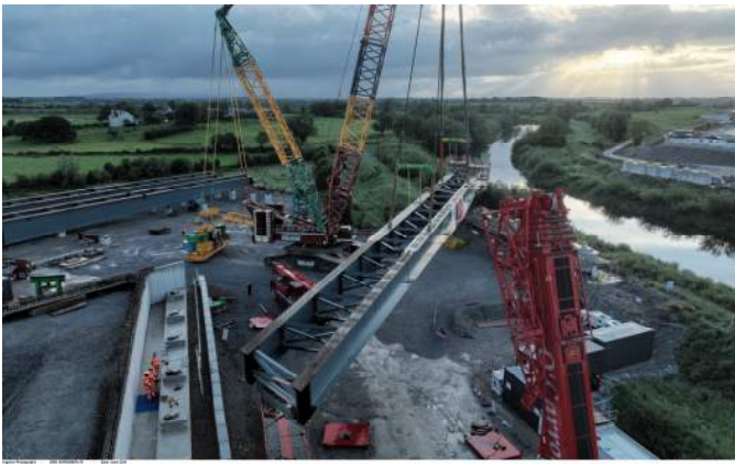
RVB04 River Bridge Steel Beam Lift
