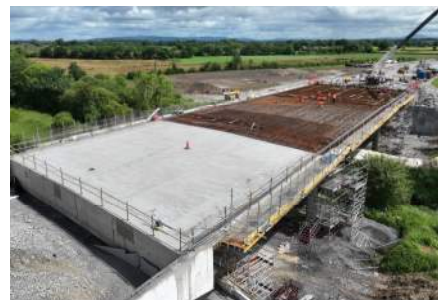
River Bridge RVB03
