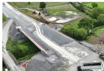
River Bridge RVB02
