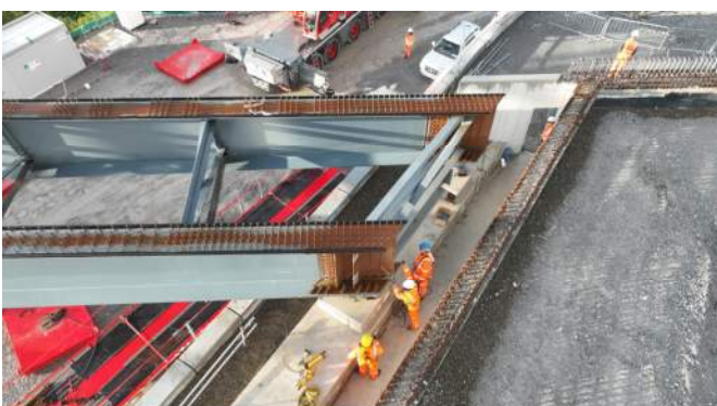
Placing Beams RVB04
